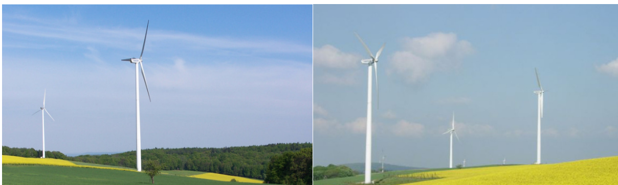
Windpark St. Wendel
